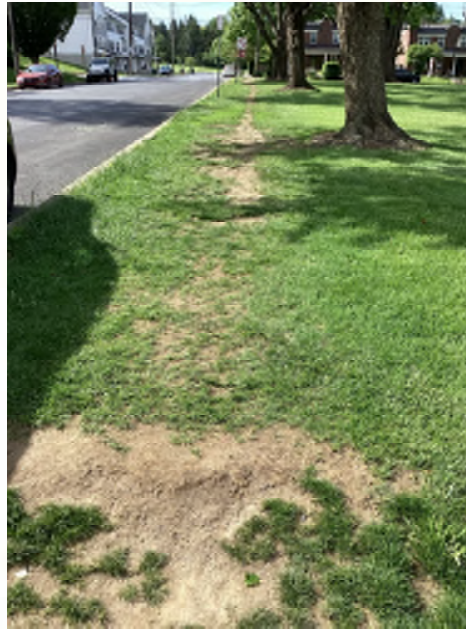
There is a lengthy stretch of missing sidewalk near the intersection of McCaskey Avenue and Madison Street.
