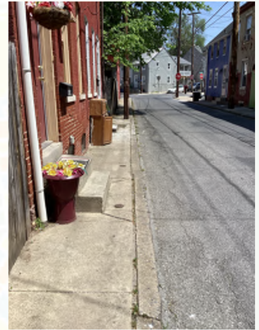
A narrow sidewalk along Andrew Street, affected by steps and a utility pole
