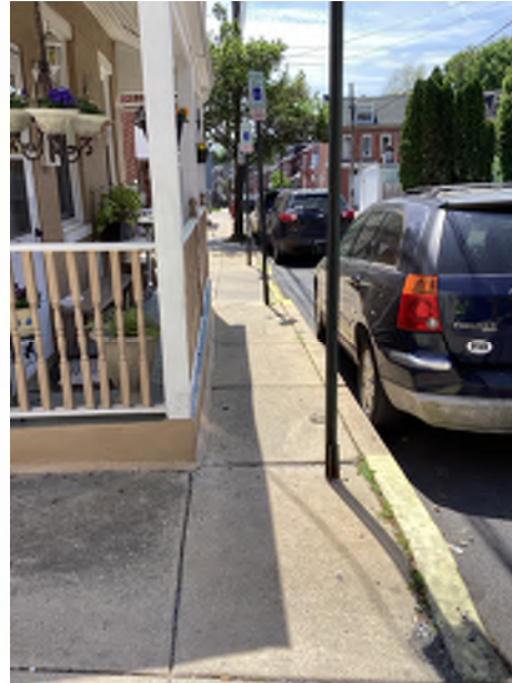
On Howard St, handicapped parking signage impedes accessibility along the sidewalk.
