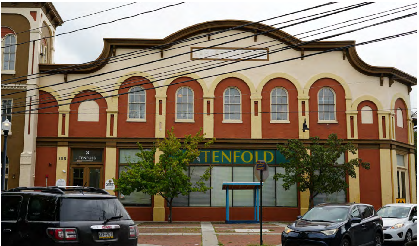
Tenfold’s comprehensive renovation/restoration of a 112-year-old TLC shelter facility (WRT)
