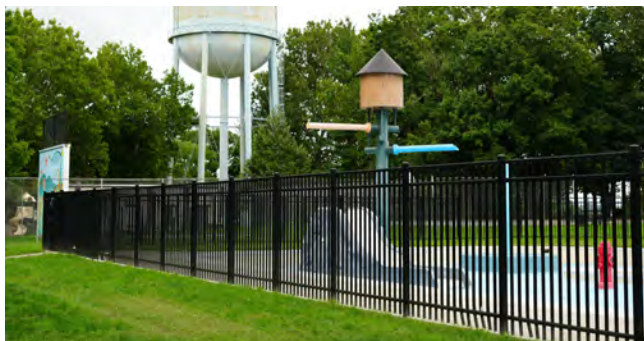
Fenced splashpad at Reservoir Park (WRT)
