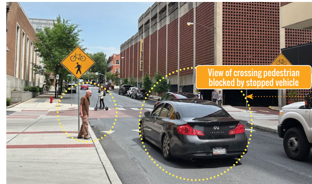
Two eastbound lanes on Chestnut Street make it difficult to see pedestrians at Christian Street
