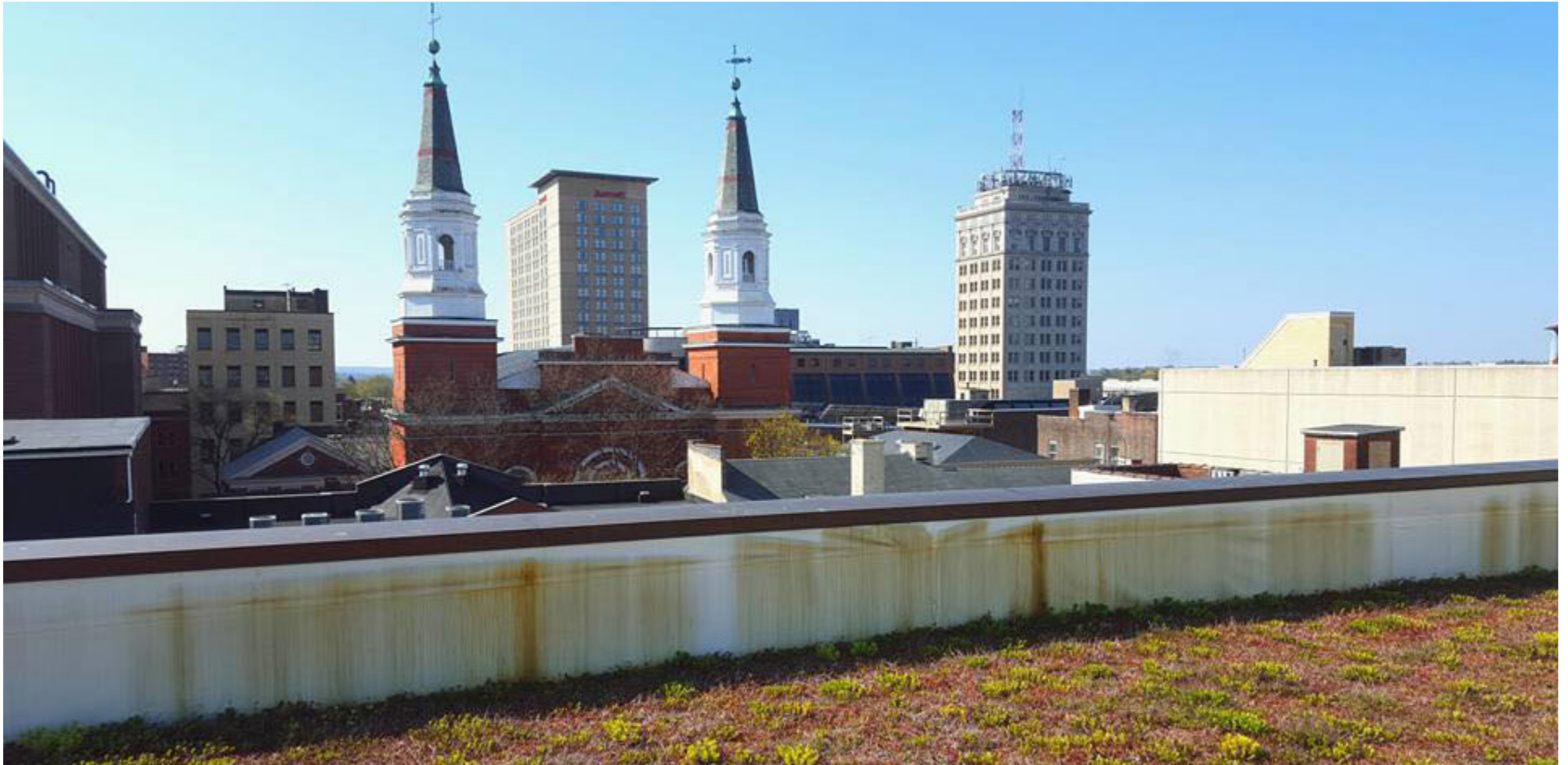
City Hall green roof.
