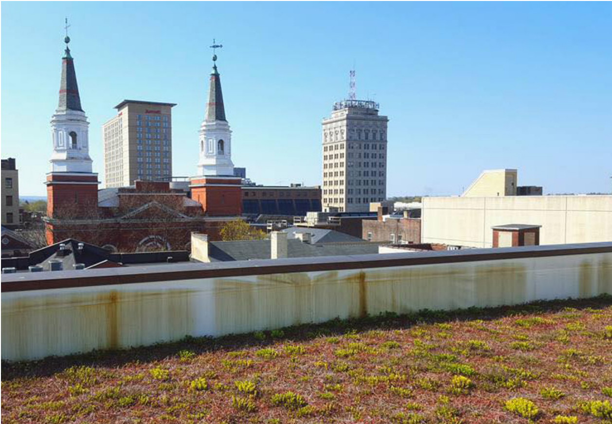
Lancaster City Hall's green roof.
